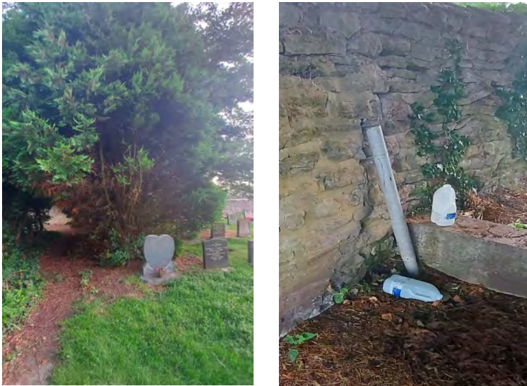
D – Water Standpipe
