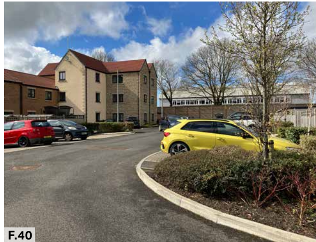
Figure 40: Recently developed 3 storey flats.
