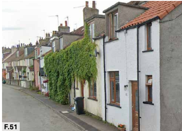
F.51 Figure 51: 2 storey housing with roof dormers in the Parkfield area.
