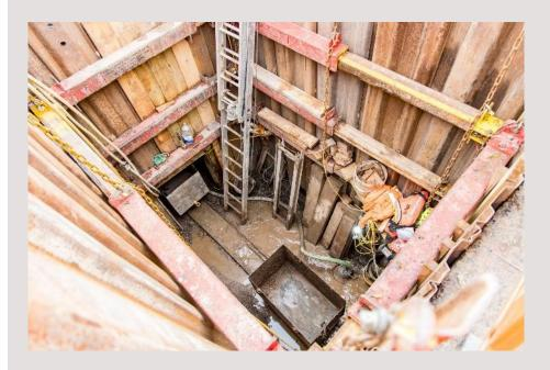
South Gloucestershire Council has been tunnelling the length of 80 metres under a section of the A4174 Avon Ring Road to replace a badly damaged drainage pipe, three metres below the road surface.
